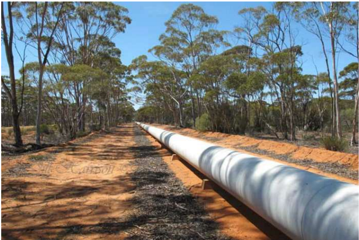
New protection pipe coatings for water transmission, both internally and externally, also acts as barrier against chemical and climatic impacts.
