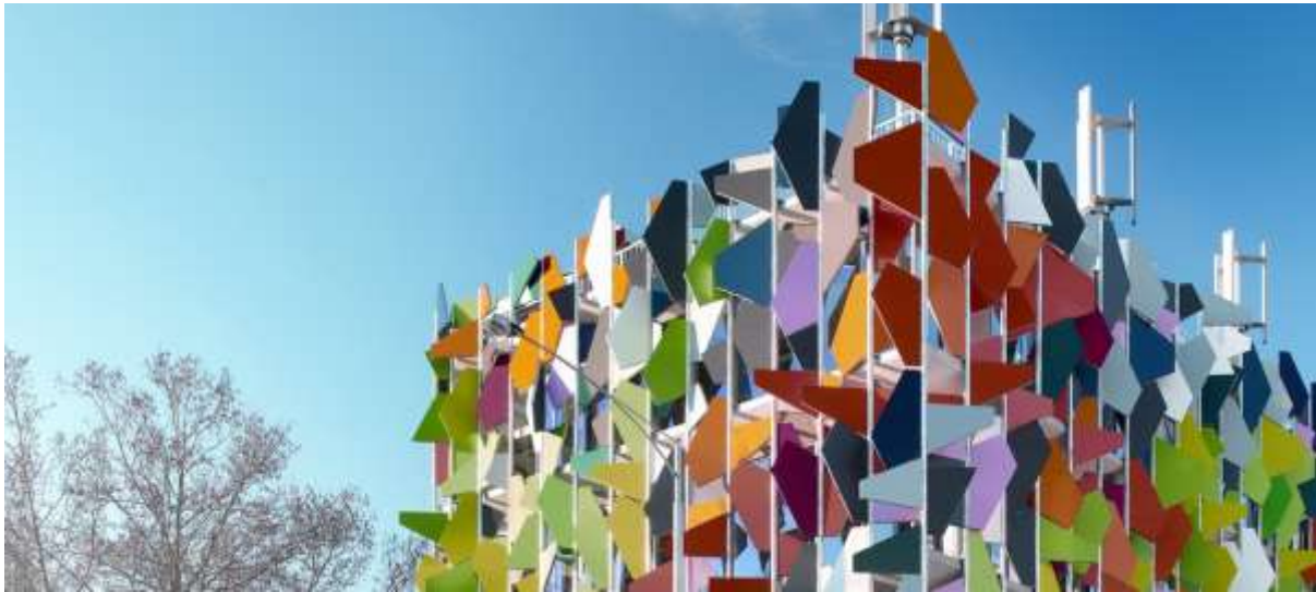
Pixel Building, Melbourne, Australia - One of the World's greenest buildings.
